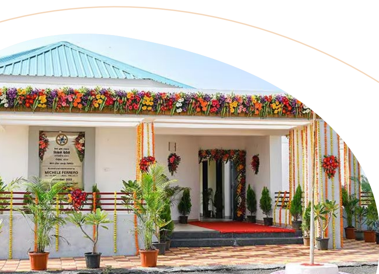
Anganwadi project, Baramati (India)
